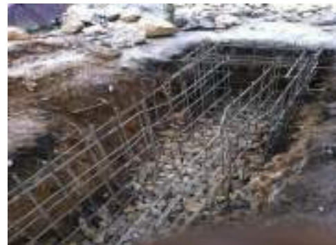
Construction of Canal
