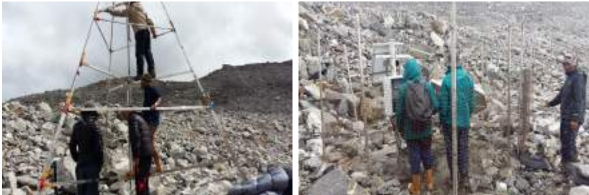
I. Assemble of Antenna of GLOF Sensor & II. Installation of Data Logger and Transmitter in South Lhonak Lake
