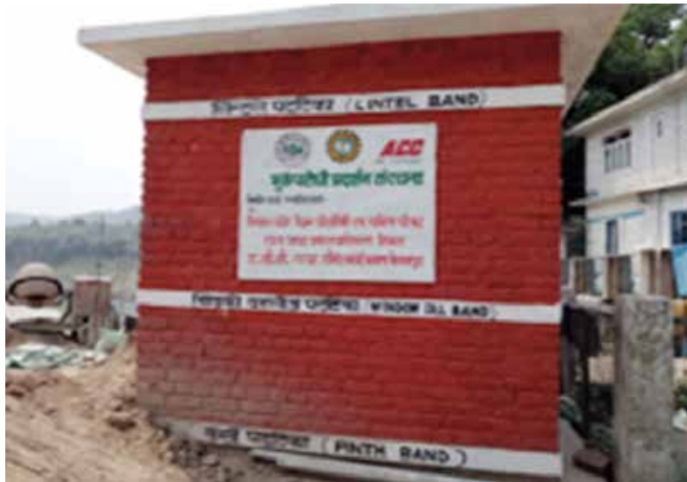
Earthquake resistant demonstration building constructed for training purpose at Dehar, Sundernagar Mandi
