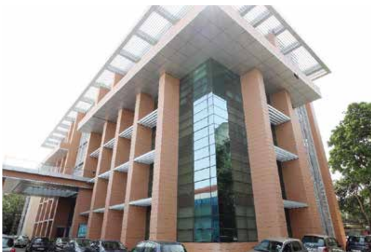
Block-II of the New State of the Art Building of Department of Science & Technology
