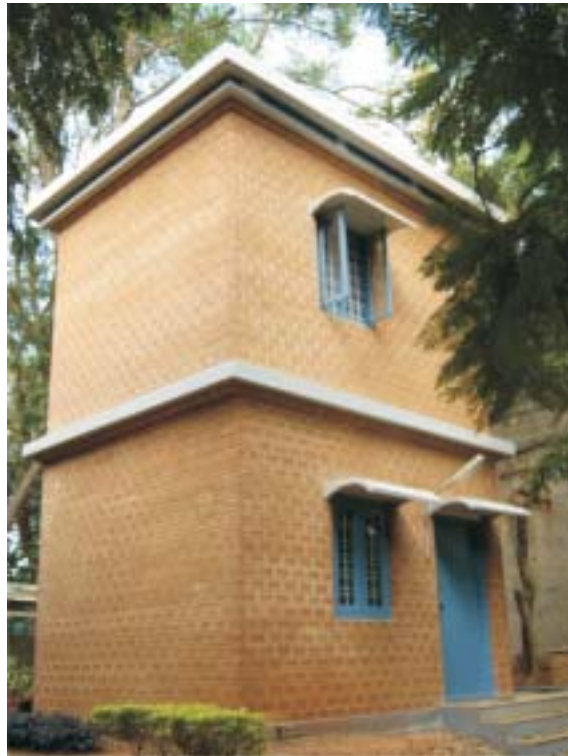
Fig. 8.8: Two storey load bearing masonry building was constructed using iron tailings as fine aggregate at IISc Bangalore.
