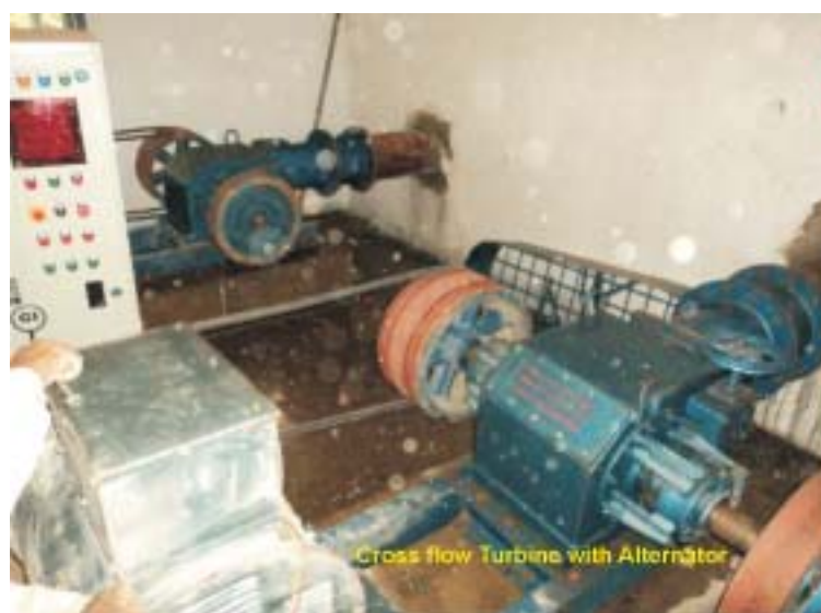
Fig. 8.6: Micro-hydel turbines at Thongleng Rong, Arunachal Pradesh
