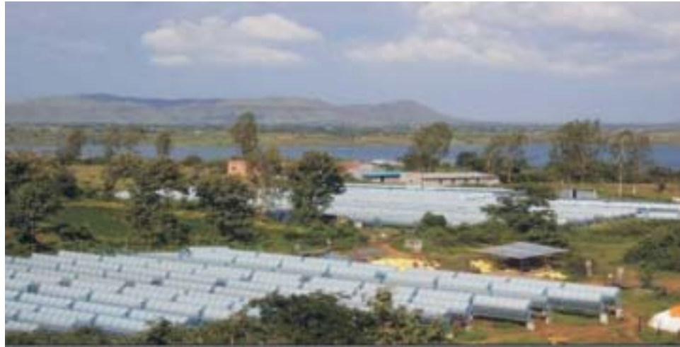
Fig. 4.38:Parabolic Trough erection & alignment completed at village Shive, Pune
