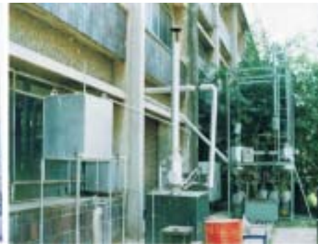
Fig.3. Fifty liter Batch capacity-Biodiesel Pilot Plant at IIT Delhi
