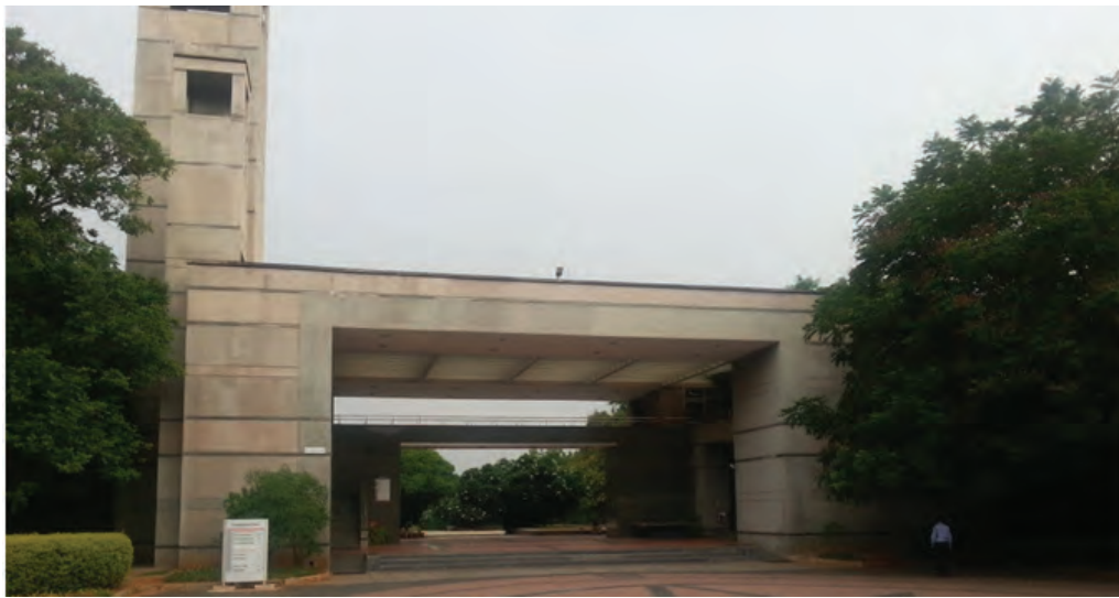
Image 1- IKP Knowledge Park main building (Source- author picture)
