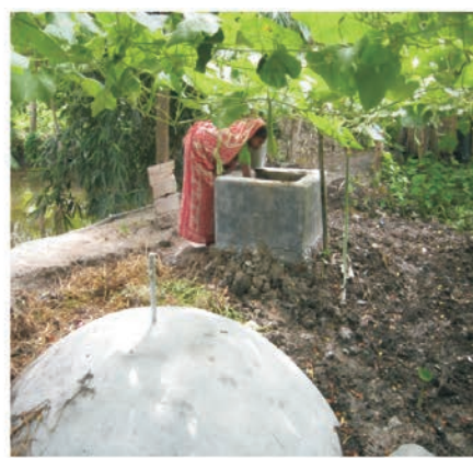
Construction of biogas plant
