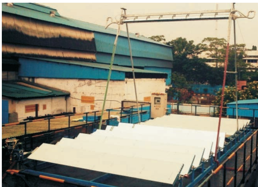
Solar-Thermal (CLFR Technology) demonstration unit at Thermax, Pune established under IGSTC project
