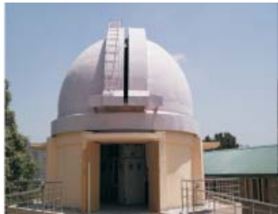
Fig. 10.5. 50-cm B-N Schmidt telescope and dome at ARIES, Nainital.
