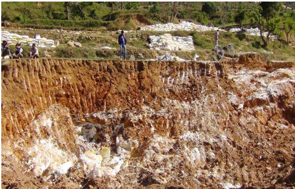
Figure 1.11. Field Photograph Showing the Removal of the Top Soil for Mining in Himalaya
