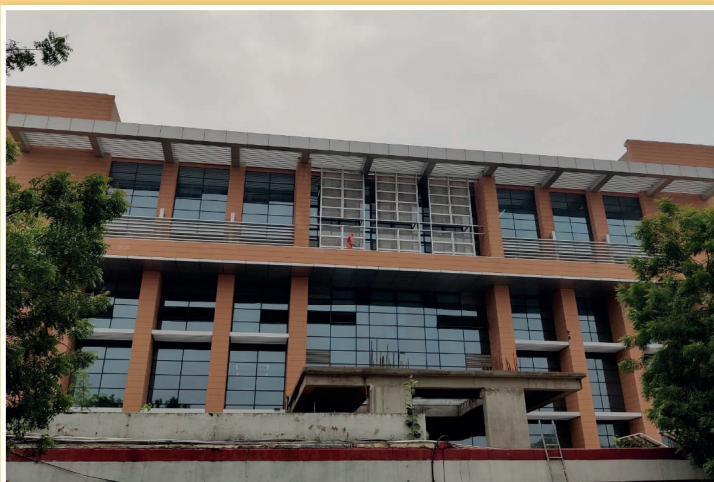
New buildings of the Department of Science & Technology
