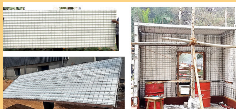
Fig. 1 Factory made EPS core panel and welded wire mesh reinforcement
